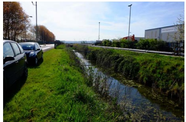
Figure 3 – Management of the existing drainage network is an important consideration
