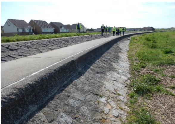
Figure 2 - A key consideration will be enhancement of the existing coastal defences
